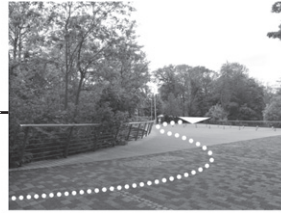
2. The bridge over the railway is transformed into a wide square, facilitating the crossing.
